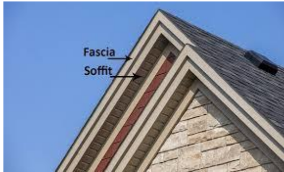
Multi-layer Fascia with a Drip Edge
