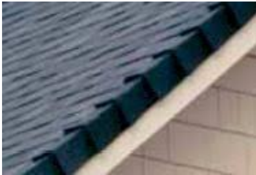
Ridge Glass on Gable Ends
